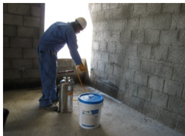
Applying DPS in the Villa
