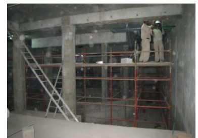
Checking the Concrete Structure
