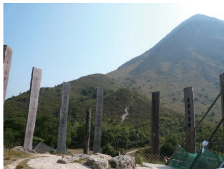
Timbers on the left hand side - treated with Everwood, Timbers on the right hand side - untreated.
