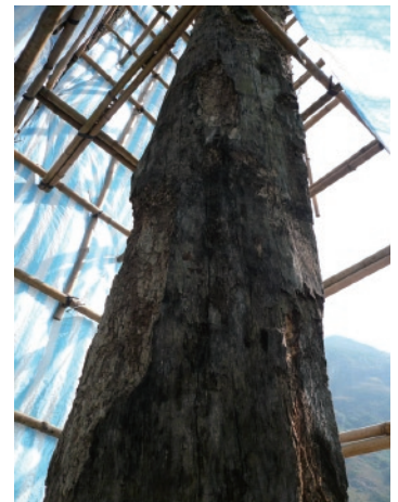
Timber column prior to Evercrete Everwood treatment.
